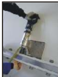
Bolting of wind tower segment with DE 15
