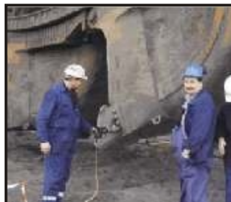
Servicing a bucket wheel excavator with a Plarad DE torque tool. No cross or impact force is transferred from tool to user
