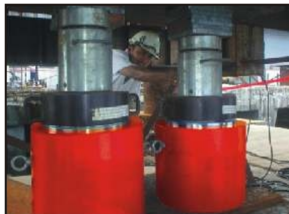
Single acting lock nut, load return cylinders used to support roof in a Tunnel Building project
