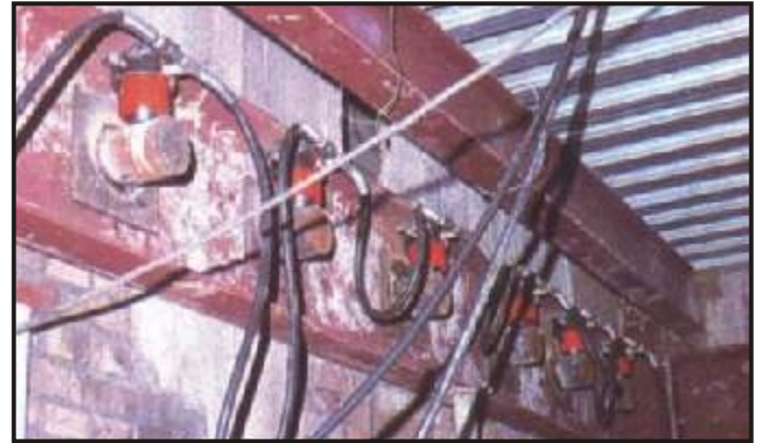
Supporting a roof during Renovation.
